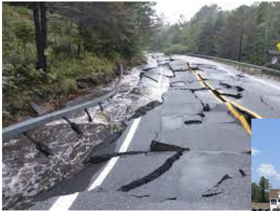
Damage to Rt. 28-N and town of Long Lake
